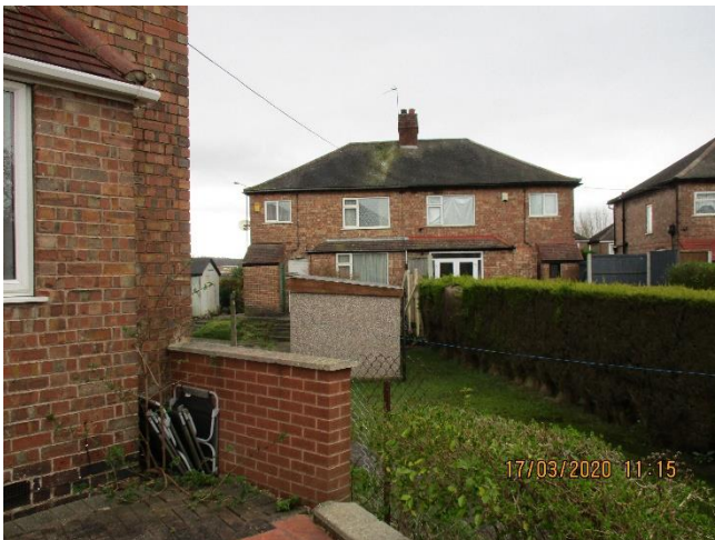
Rear boundary with no. 316 Queens Road.
